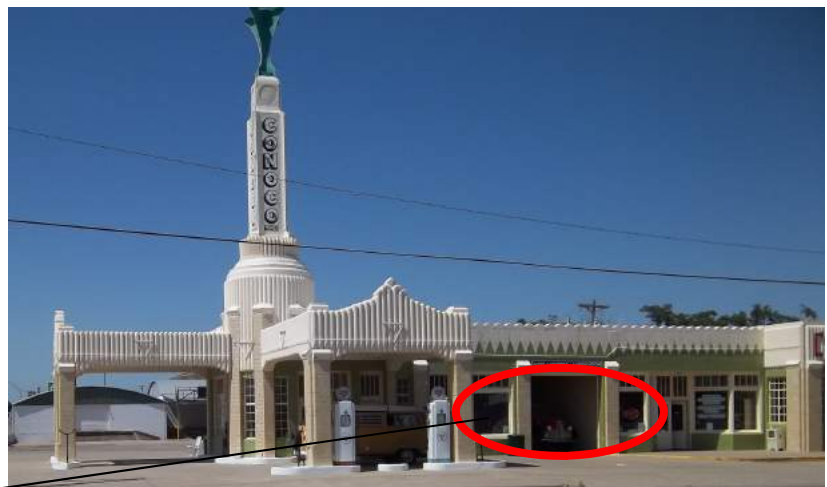
Photo on left shows the detail of the circled area in the photo above. The M truck is parked in the lube and car wash garage of this old Conoco station, now a museum, built along Route 66 in 1936.
